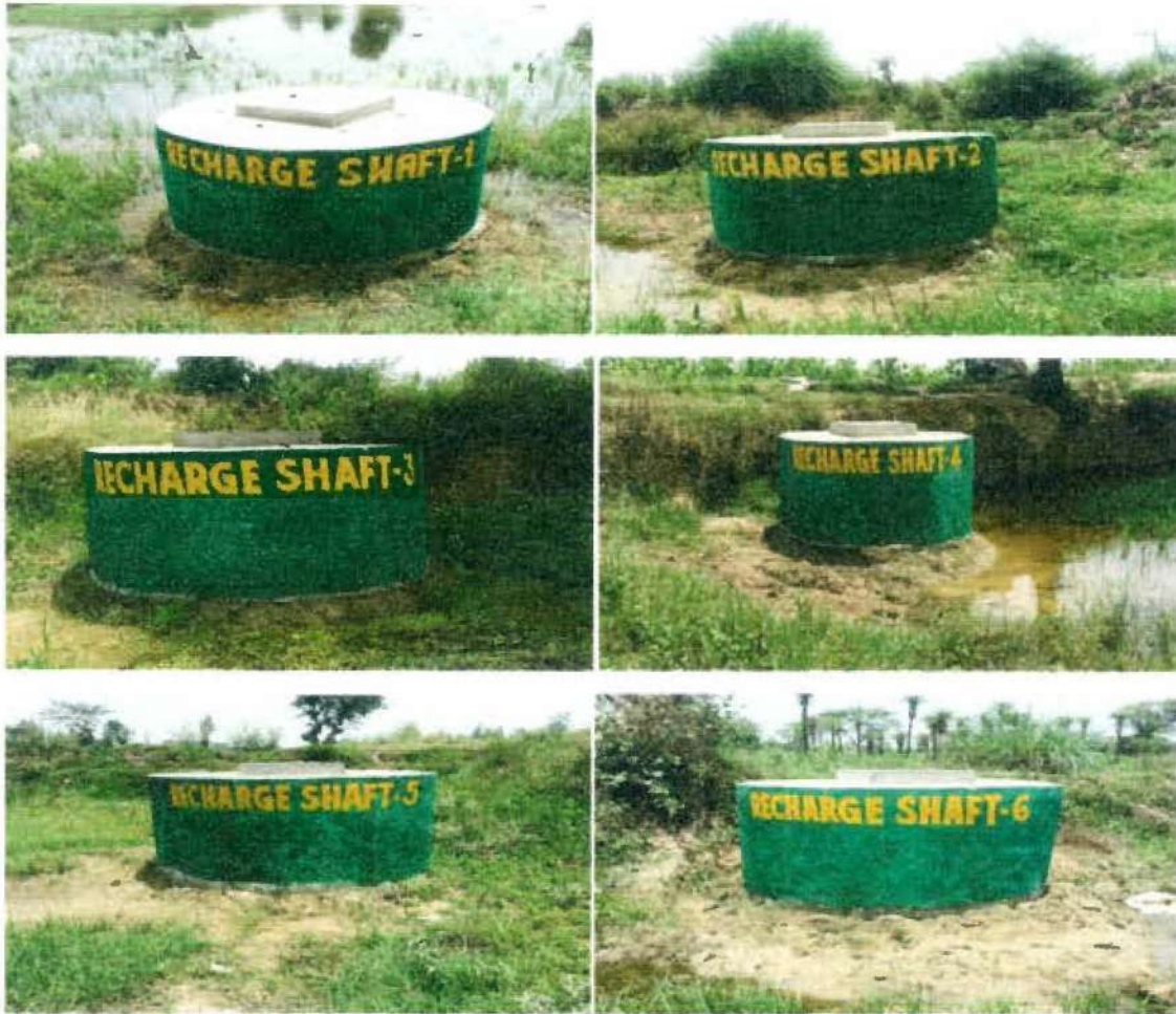
Fig 17: Photographs Showing Construction of 6 Recharge Shafts in Pond of Nagla Mubarik
