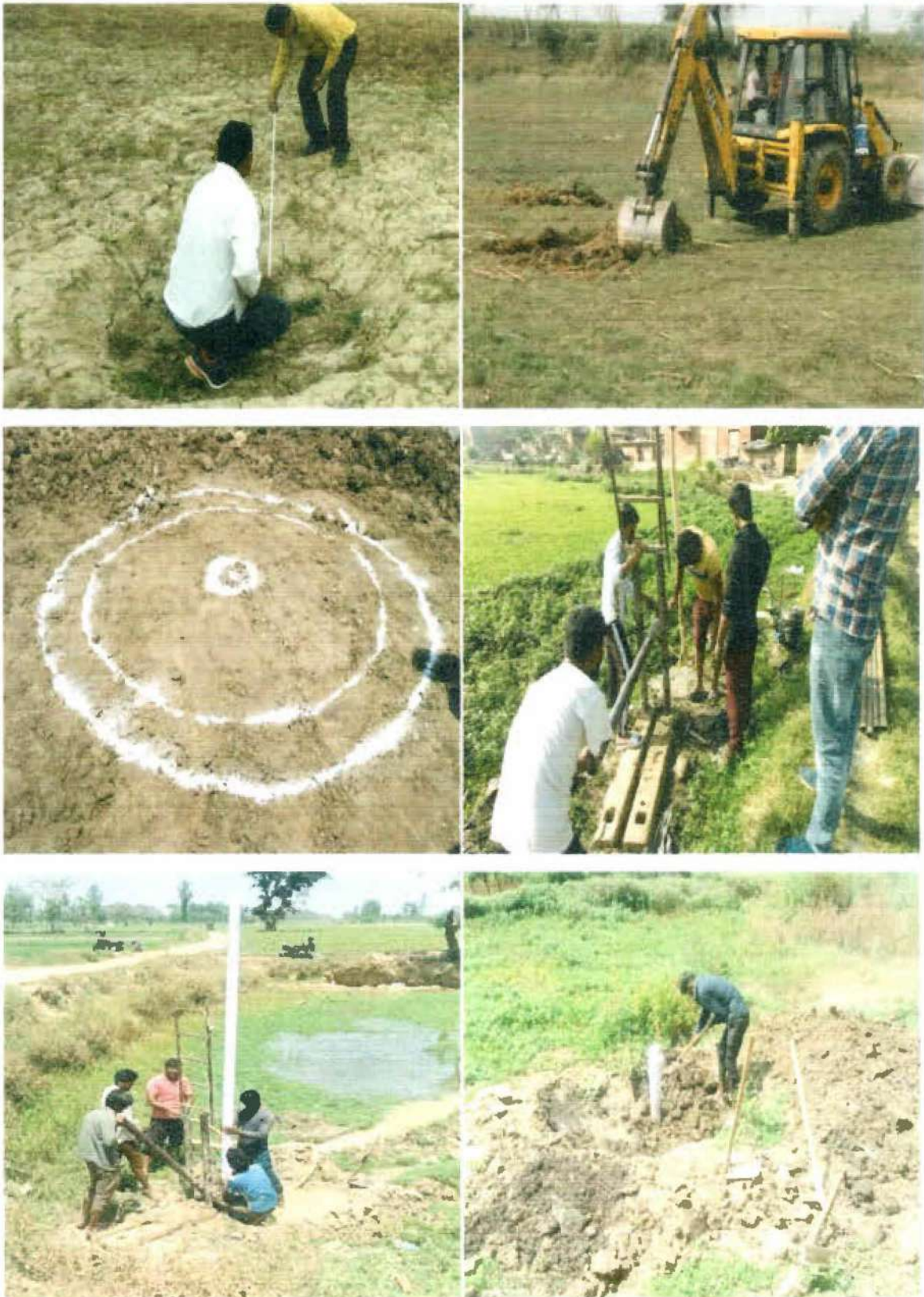
Fig 16 a: Photographs Showing Survey and Construction Work of Recharge Shafts
