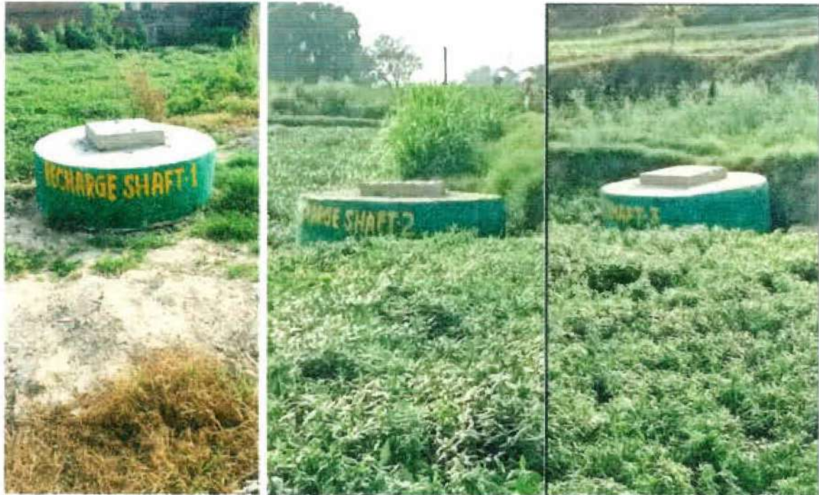
Fig 25: Photographs Showing Construction of 3 Recharge Shafts in Pond of Bhikki
