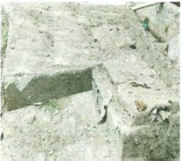
RWH -6 Location: Cooling Tower Geolocation: 29.427271, 77.761330
