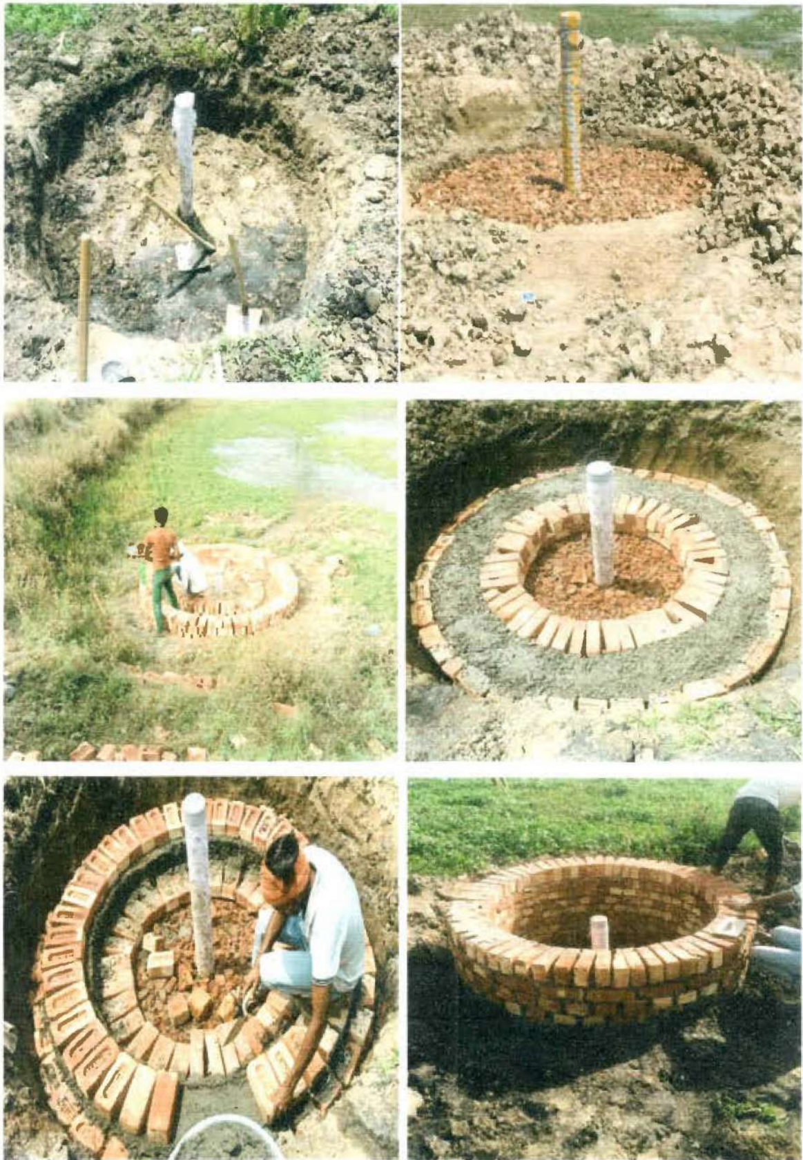
Fig 16 b: Photographs Showing Survey and Construction Work of Recharge Shafts
