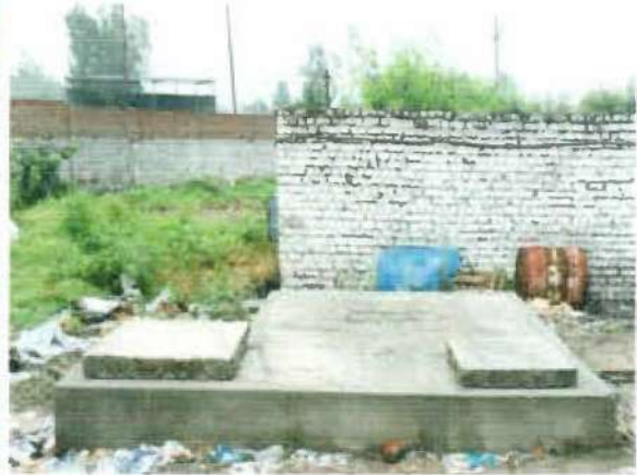
RWH -2 Location: Backyard unloading Geolocation: 29.426000, 77.763673
