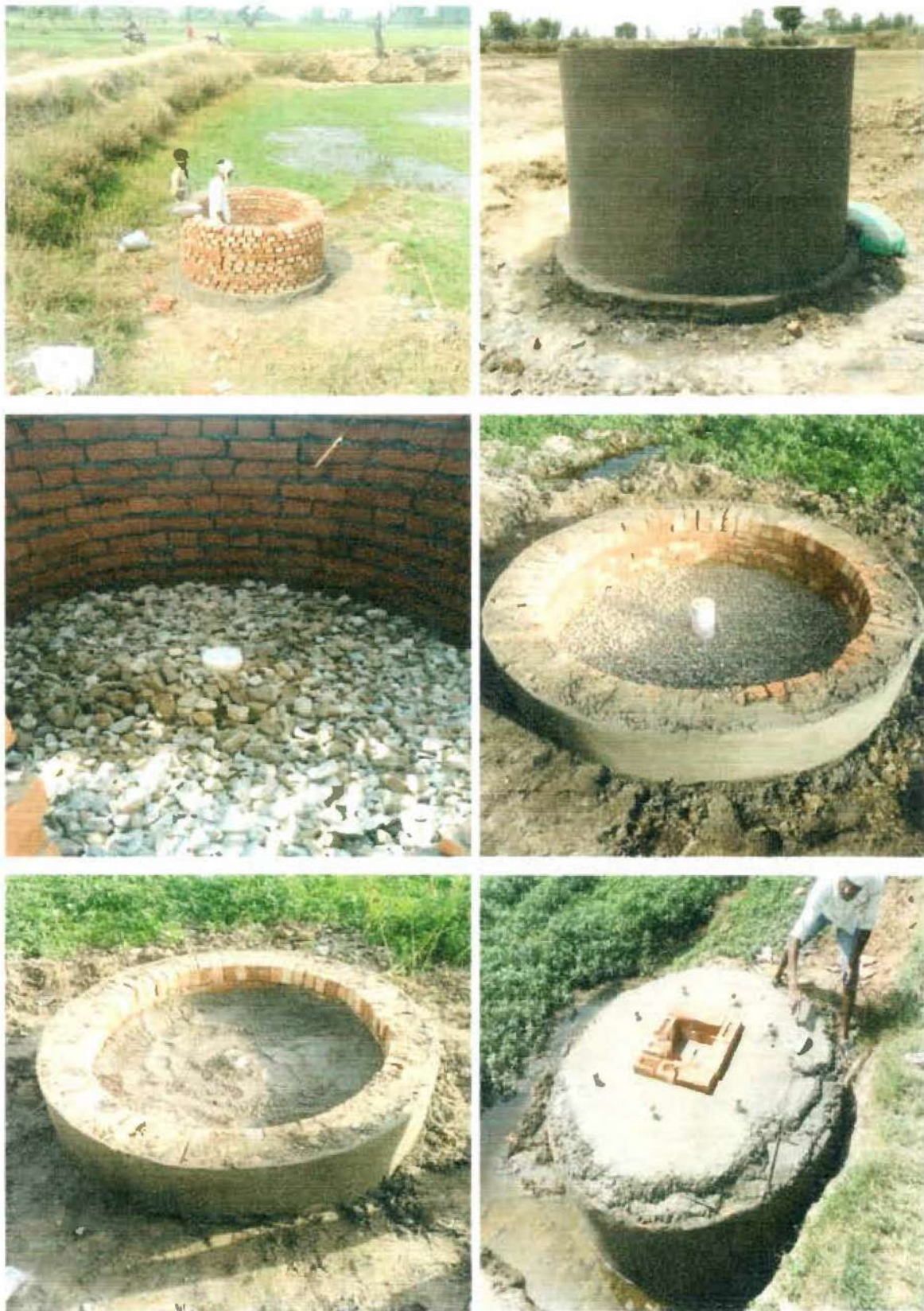
Fig 16 c: Photographs Showing Survey and Construction Work of Recharge Shafts
