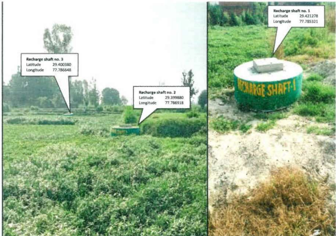
Fig 26: Photographs Showing Geo-Location of Recharge Shafts in Pond of Bhikki
