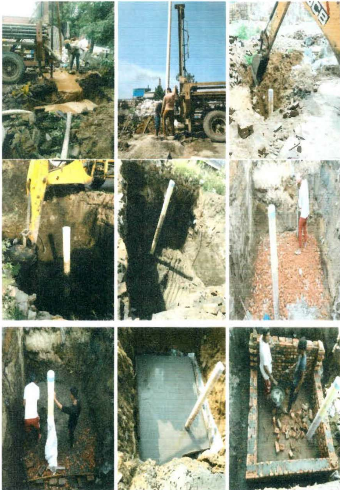
Fig 14a: Photographs Showing Construction of Rainwater Harvesting in factory campus
