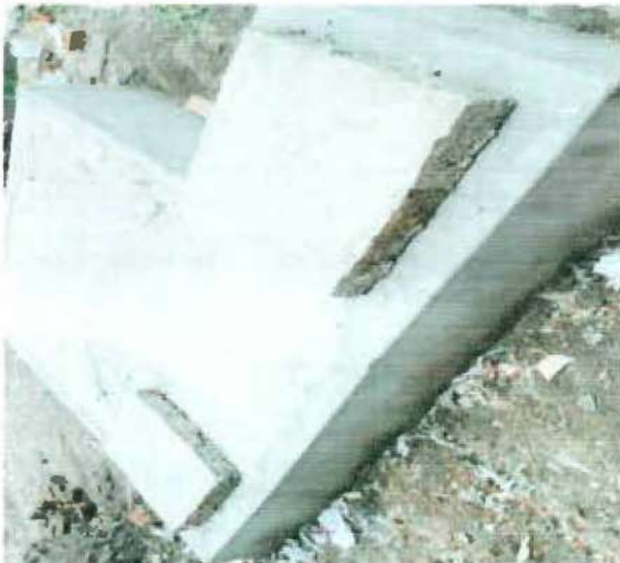
RWH -5 Location: Brown paper Processing (PM-2) Geolocation: 29.427053, 77.761393
