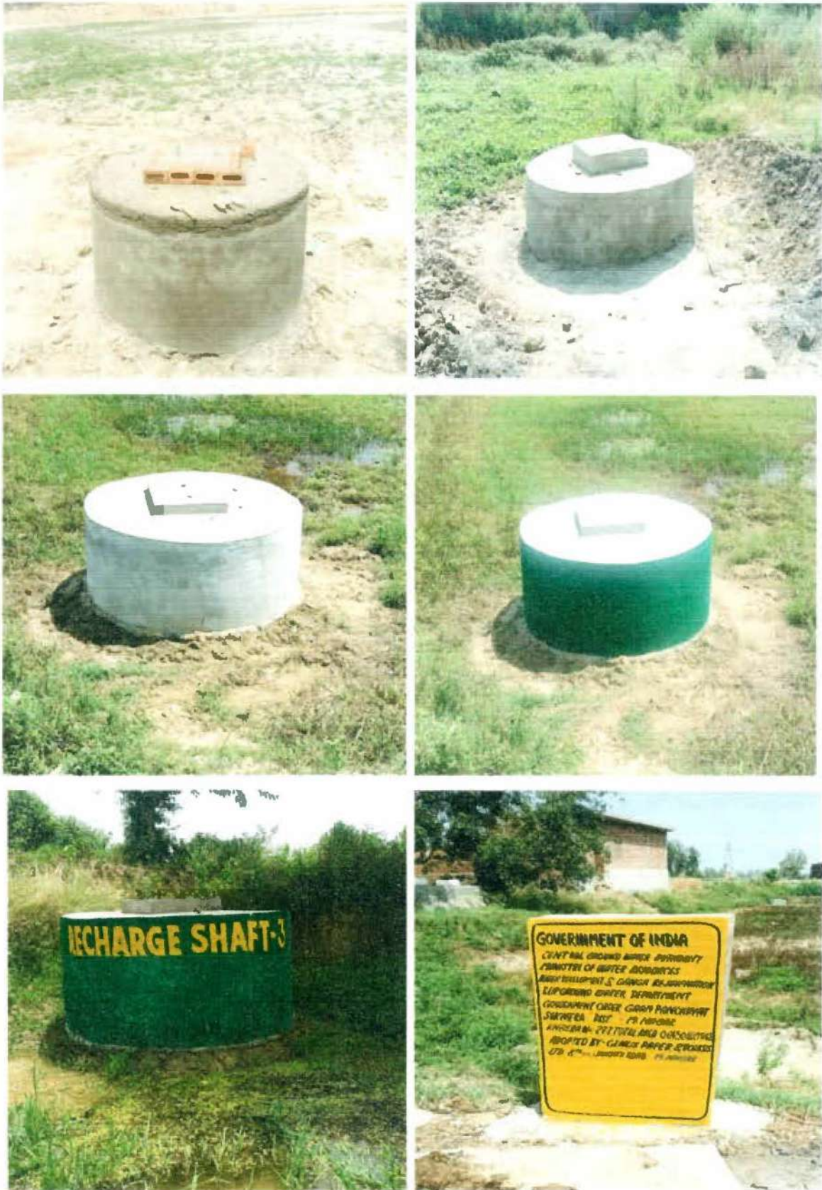
Fig 16 d: Photographs Showing Survey and Construction Work of Recharge Shafts
