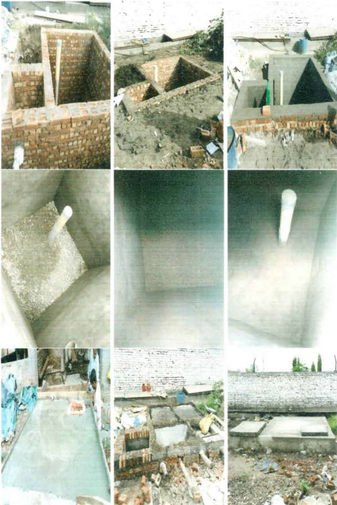
Fig 14b: Photographs Showing Construction of Rainwater Harvesting in factory campus
